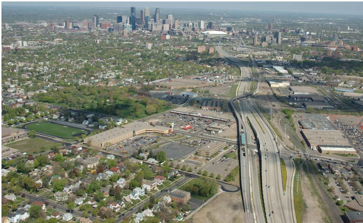
The Hiawatha – Lake intersection and Midtown LRT station area, looking northwest.
